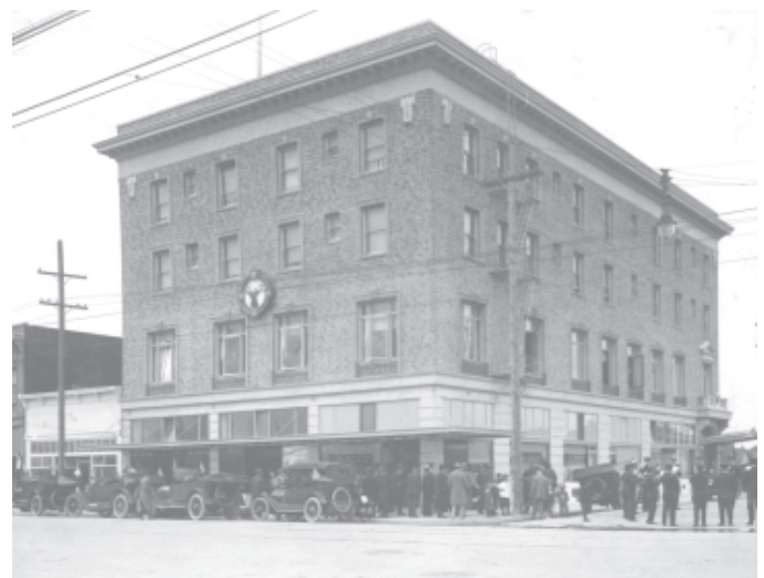
The Elks Building, 10 th St. & Macdonald Ave. ca. 1916.
